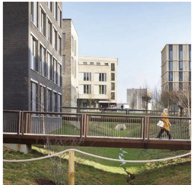
SUDs incorporated into the residential landscape
