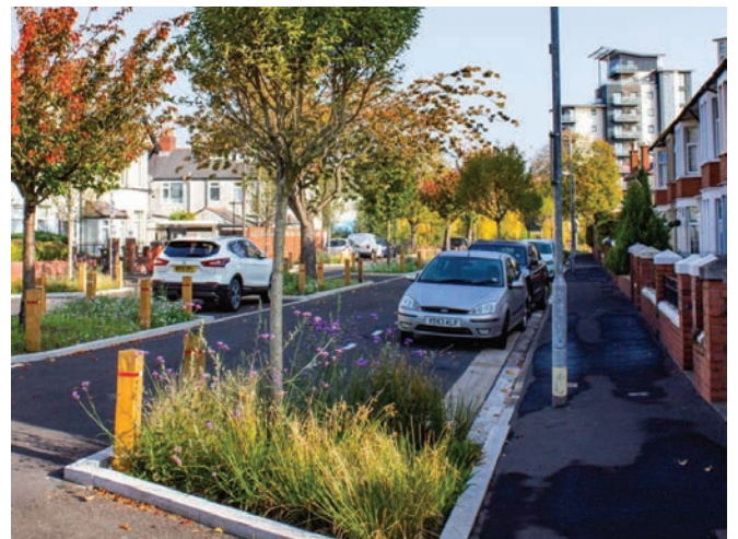
Bio-retention tree pits
